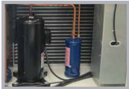
scroll compressor many of the NDX (models NDX 0250 (460/3/60) and up) utilize scroll compressors. Scrolls minimize power consumption, noise, vibration and moving parts while maximizing reliability and resistance to liquid refrigerant returns
