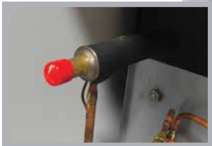
automatic expansion valve the TXV ensures stable dew point performance even in changing ambient conditions
